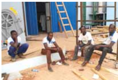
INSTALLATION / Safi Sarl
